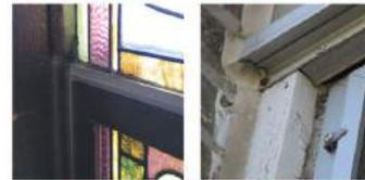
Example of interior & exterior ventilator window frames
