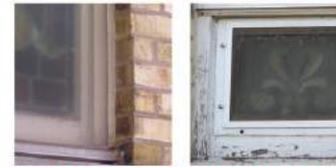
Example of exterior frames with storm glass and screen
